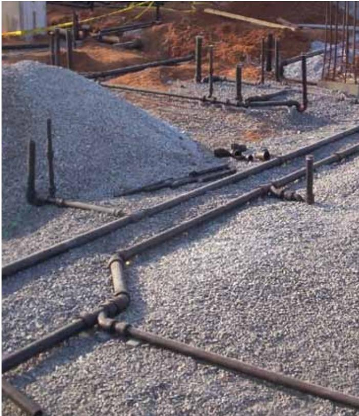
Cast iron soil pipe expands 3/4 in. per 100 ft. per 100° F change (approximately the same as concrete). As a result, thermal expansion is not typically a concern with cast iron soil pipe systems.
