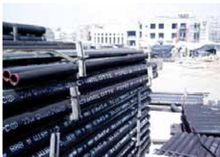
Cast-iron piping is a cost-effective solution when dealing with fire-resistive construction because it will not melt or burn away in a fire.
